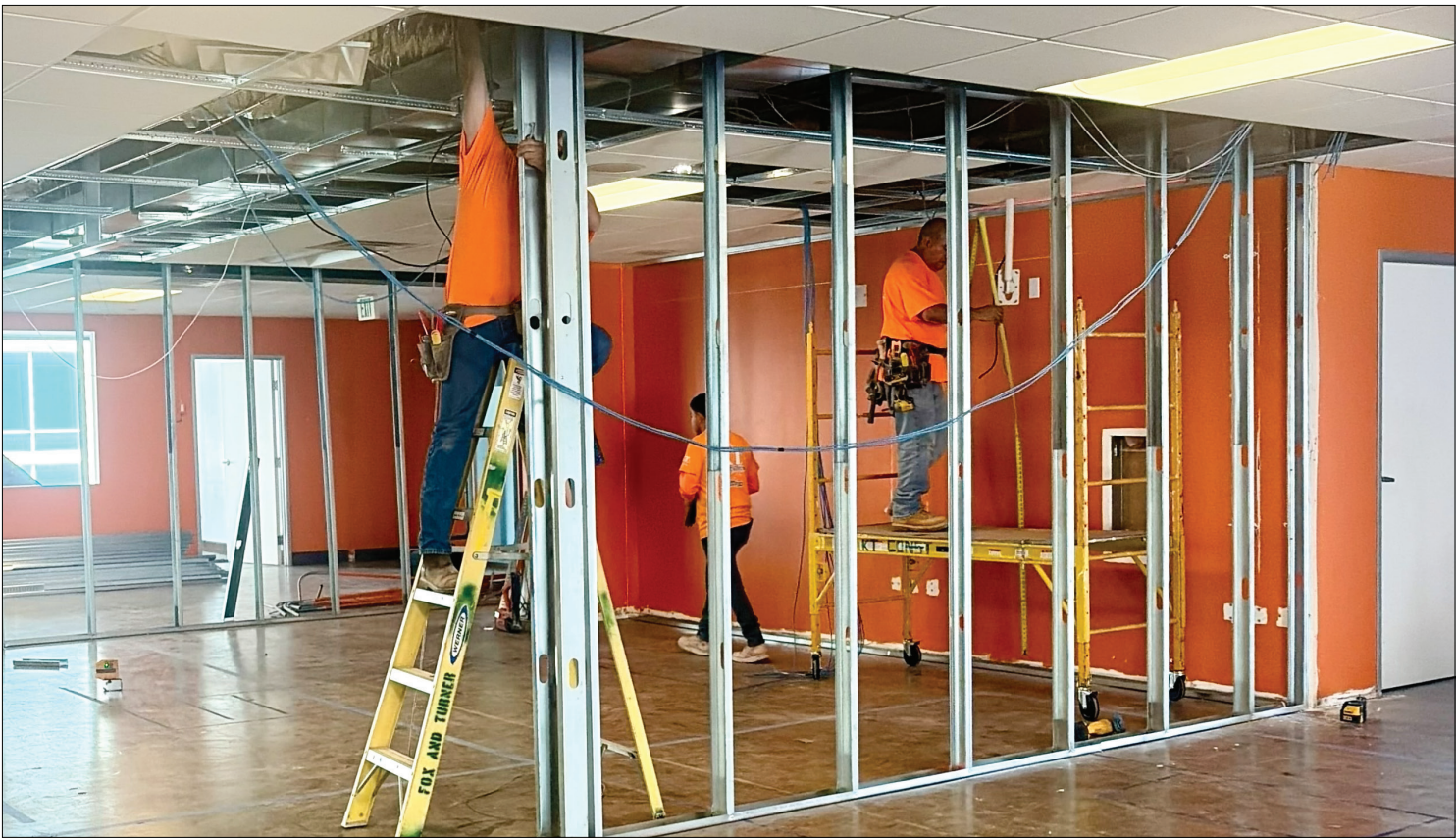
Outside The Lens is renovating the fifth floor of 925 B St. as its new home. Photo courtesy of Outside The Lens
